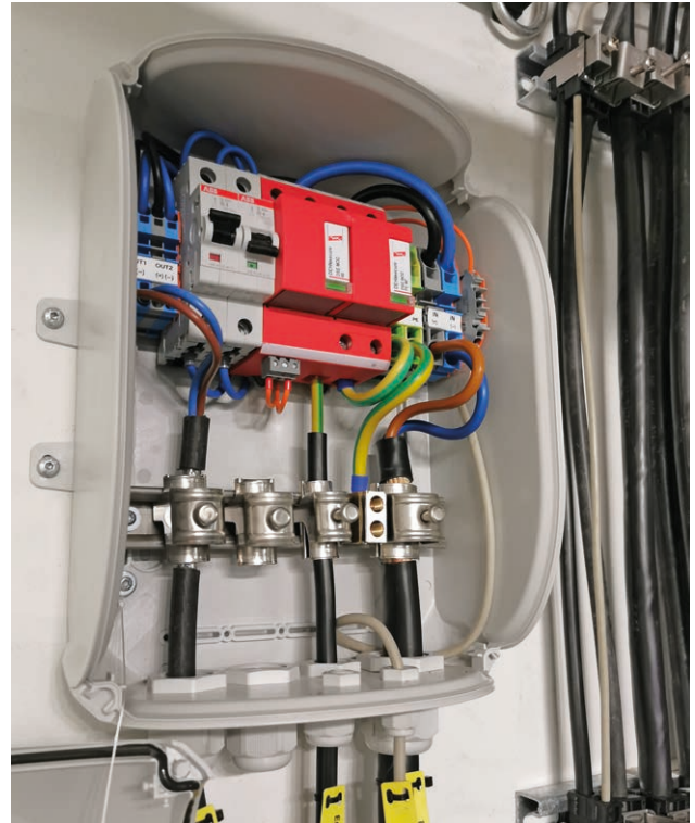
Protection of the voltage supply of a mobile radio transmitting system by means of the DEHN OVP box
