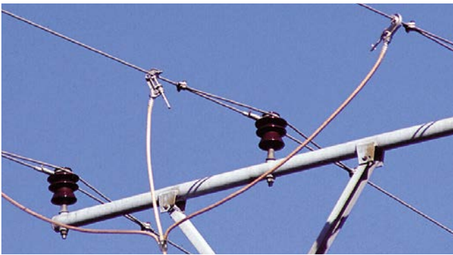
Phase screw clamps used on an overhead line
