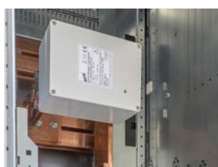
Built-in quenching devices
