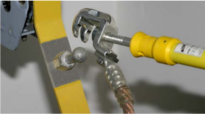
Connecting the phase cable end with universal clamp to a fixed ball point
