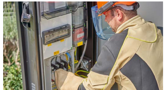
Maintenance of charging posts.
