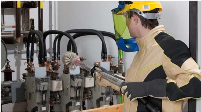
Live cleaning of a transformer using the TRS MS dry cleaning kit.
