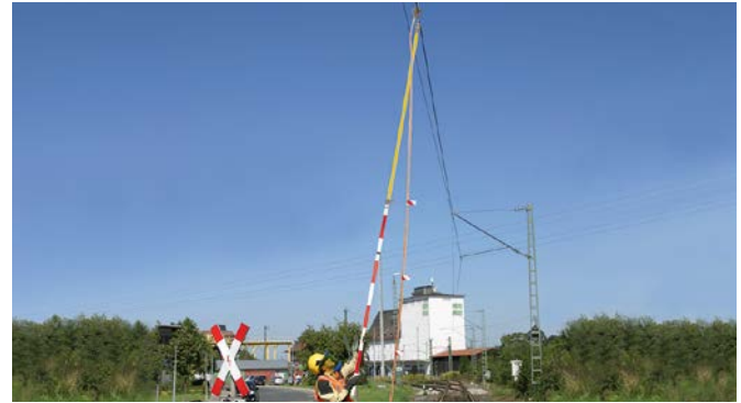
Attaching a railway earthing device.
